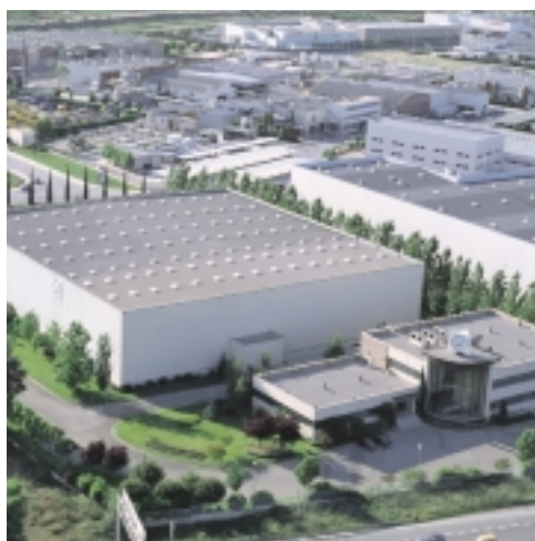
Commercial offices and end product warehouse.
